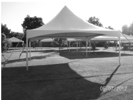
20 x 20 frame push pole tent. Note the staking.
