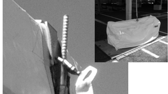
The tensioner is not a proper connection point for clearspan, the 3,200 lbs. block is not enough to ballast this tent. This company lost this very same tent in a 45 mph wind.
