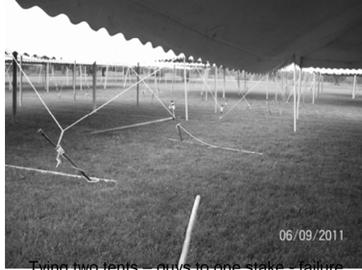
Tying two tents – guys to one stake - failure
