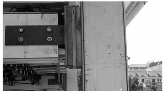
Improper install - not a 2 story tent, upright bent under stress. Undersize bolts, shimmed gap with wood.
