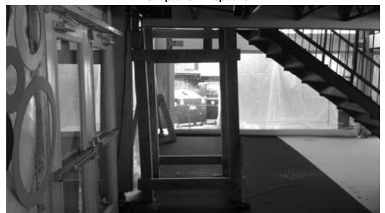
Emergency stair case - exit. What's wrong with this?
